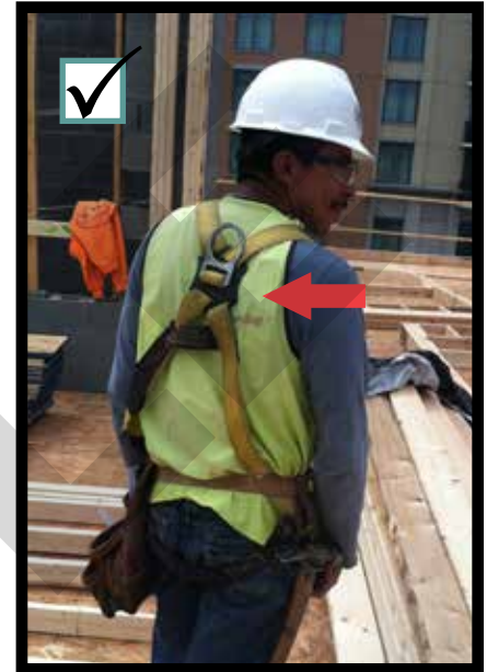
D ring should be located between shoulder blades. El anillo D debe localizarse entre los hombros.
